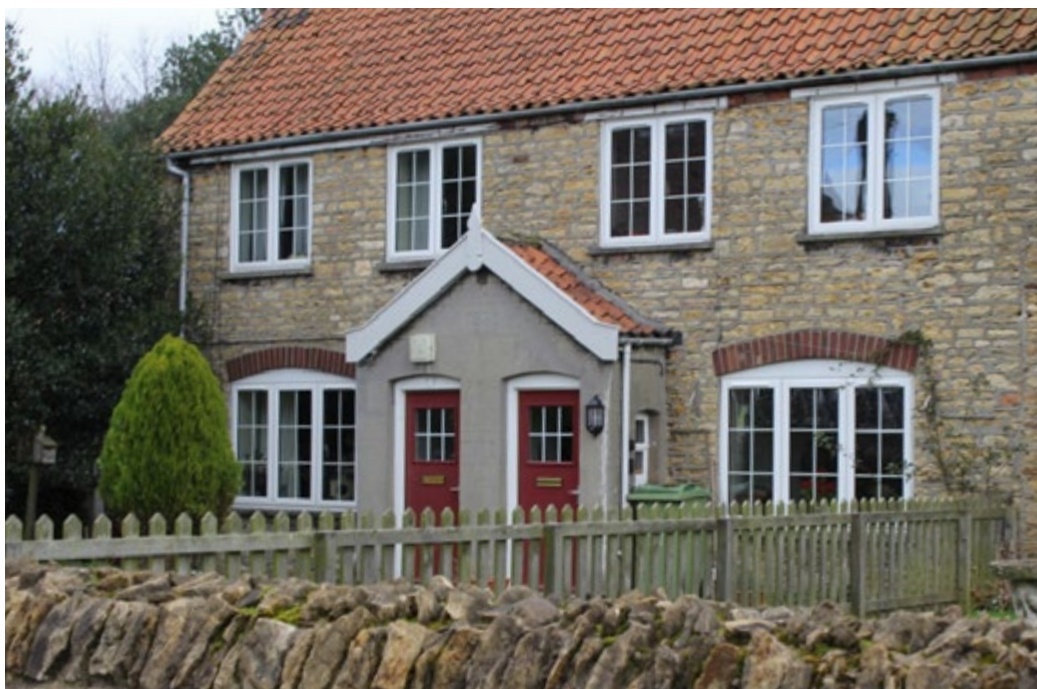
Left: Housing in Willoughton showing the distinctive combination of limestone walls and boundaries, red clay pantile roofs and red painted front doors.
